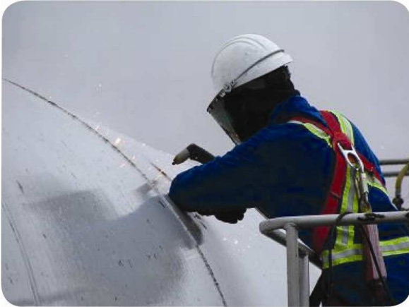
The first of many cuts made to the bullet tanks
